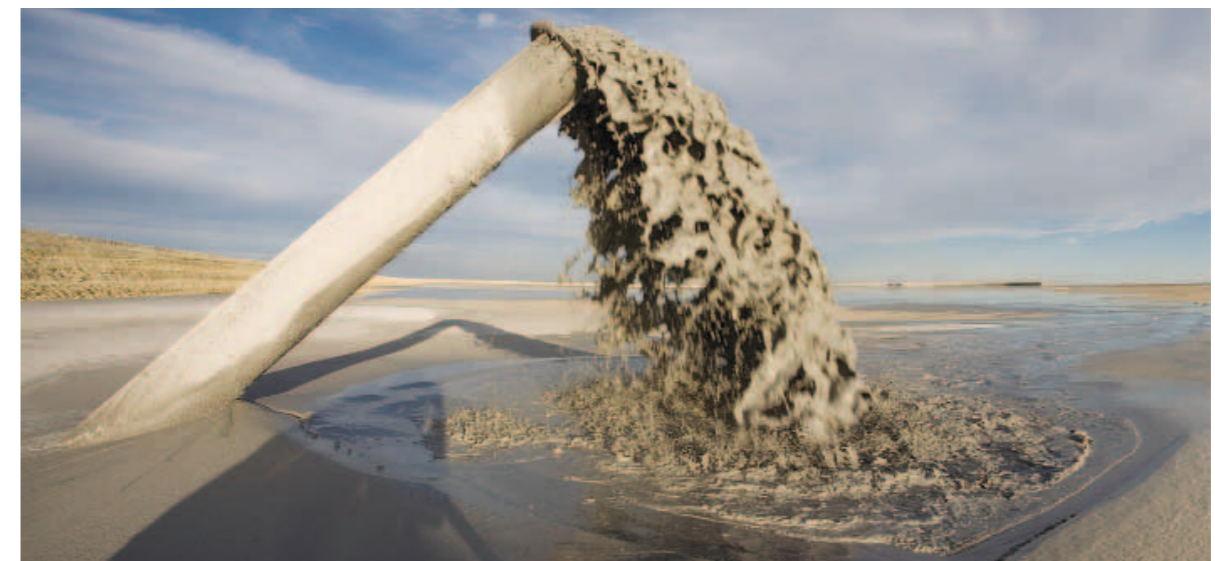
Tailings discharge. Stefanutti Stocks Mining Services originally made its name as a specialist designer, constructor and operator of tailings facilities and this remains a major part of its business.
