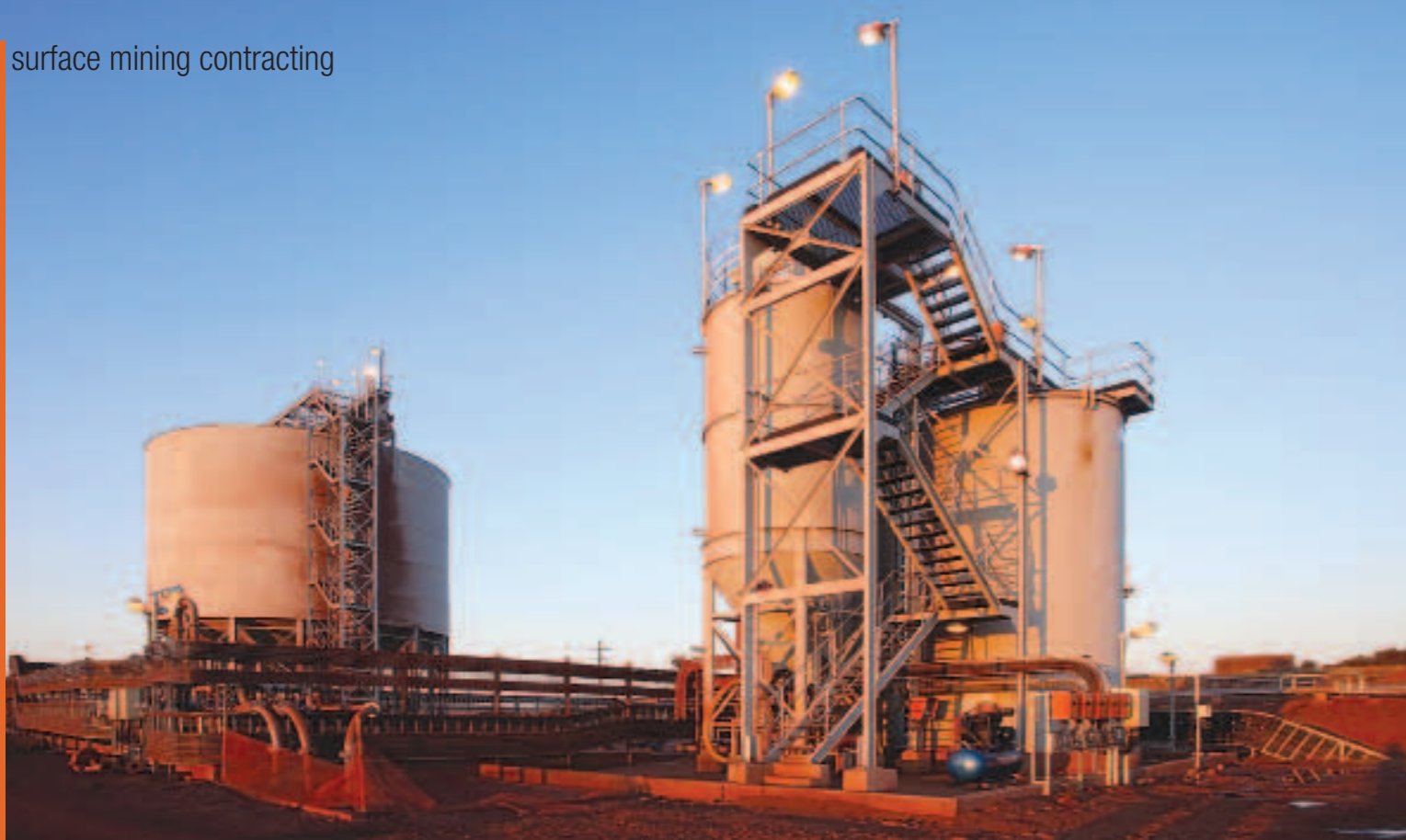
A paste thickener plant. Stefanutti Stocks Mining Services is one of the pioneers of this technology in South Africa.
