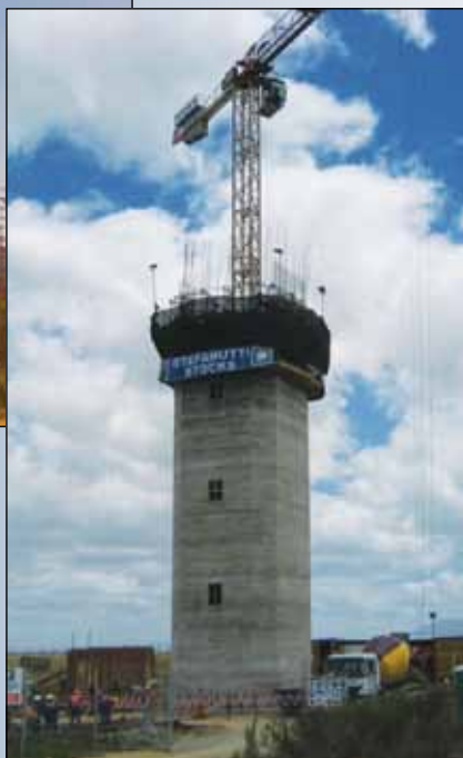
Slipforming the shaft and lifting the external platforms of the George Airport radar tower.
