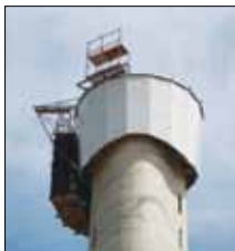
Traffic control tower at Sikhupe International Airport, Swaziland.
