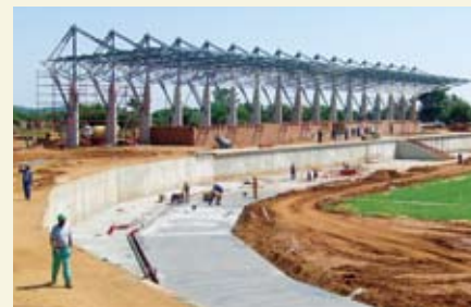
The Moruleng Stadium is progressing well.
