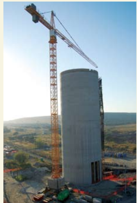
The Amandelbult Silo, completed in 2008.
