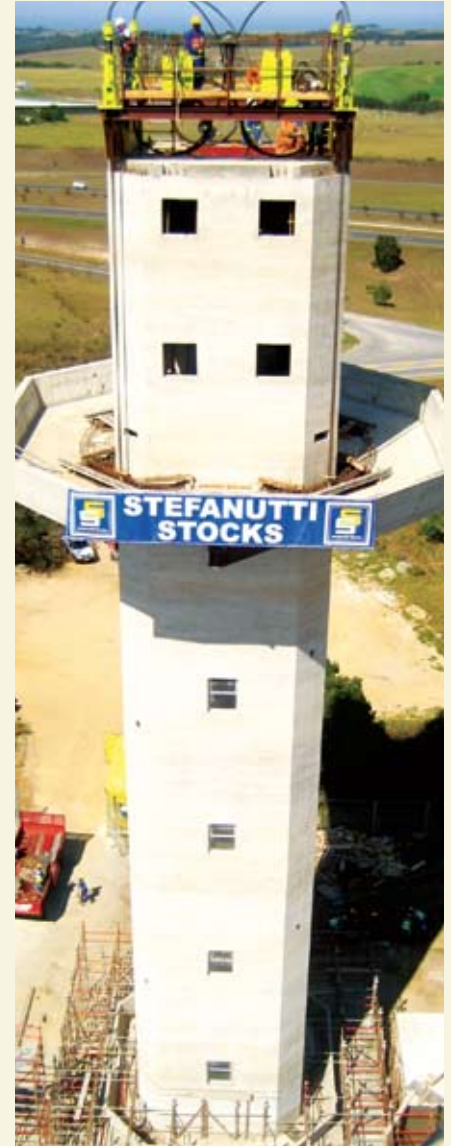
The George Radar tower, under construction with platform lifting in progress.
