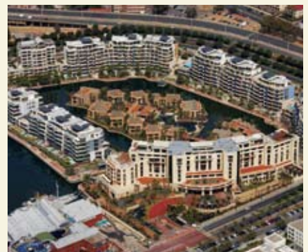
An aerial view of the entire development including the hotel, the two man-made islands and the canal system surrounding the luxury hotel.
