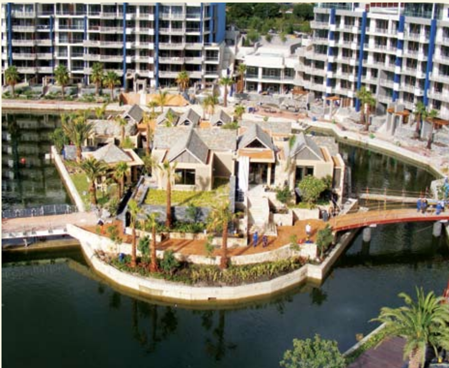
On one of the two man-made islands in the V&A basin a state of the art luxury spa facility has been constructed as seen above. Visible on the left hand side is the bridge linking the spa island to the second island which has an open air restaurant, resort style heated swimming pool and 11 luxury villas with a total of 40 guest units. The mainland and islands are linked via bridges and tunnels below the canals.
