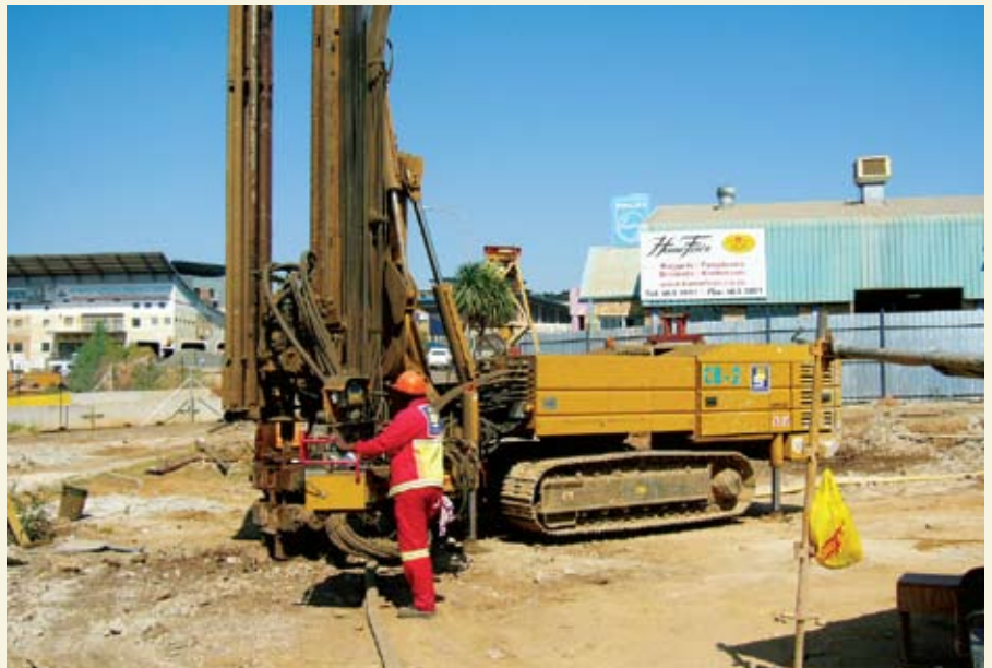
CB crawler rig in the dolomites.
