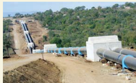
The 780m long invert siphon.
