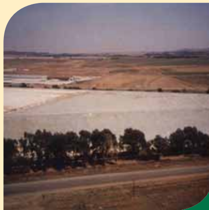
View of completed dam portion.
