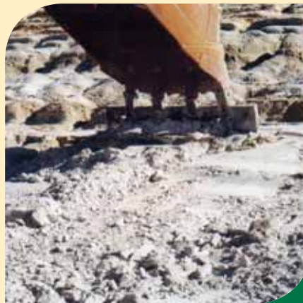
Preparation of the slope with a modified excavator bucket.
