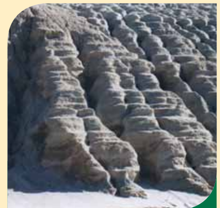
Typical erosion to untreated side slope of a tailings dam.
