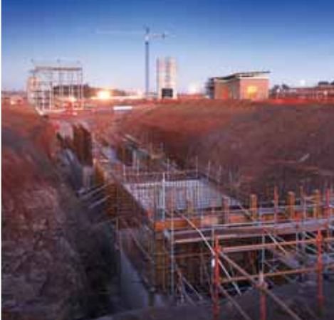
The circular stacker under construction.
