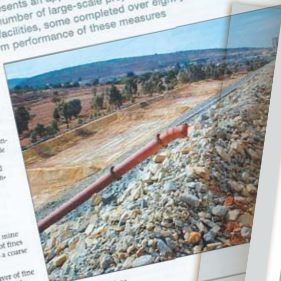
A completed side slope
