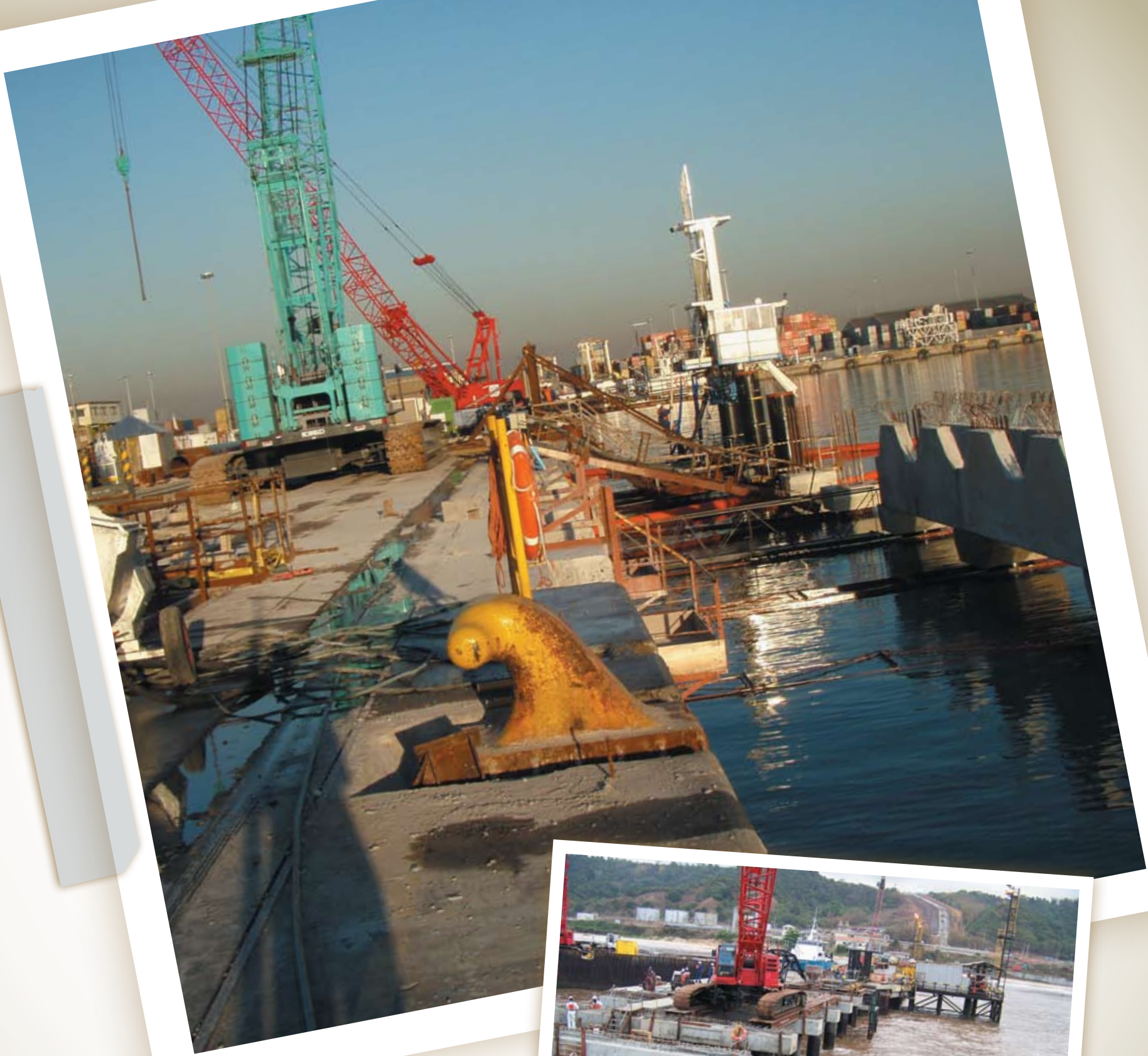
Ben Schoeman Dock construction congestion!
