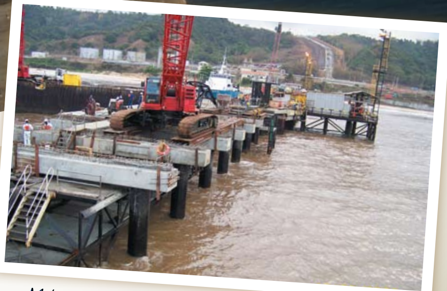
Malongo Dock expansion.
