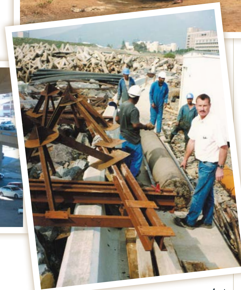
Greg at Granger Bay concrete works - the first project for Entech.
